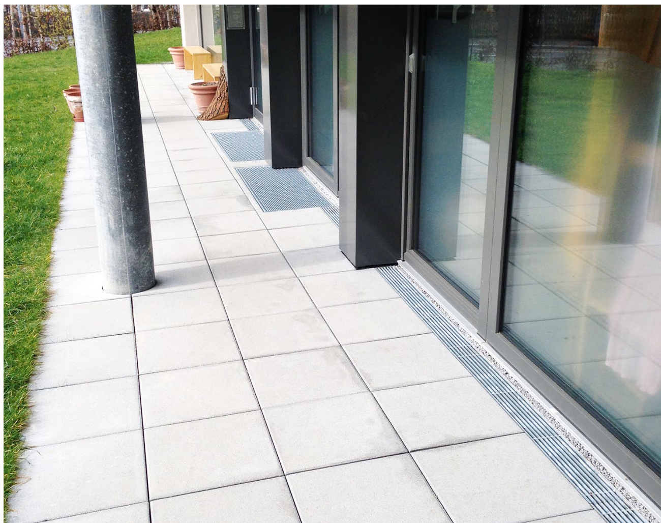
Residence hall Scheuchzerstraße, Zurich, Switzerland
