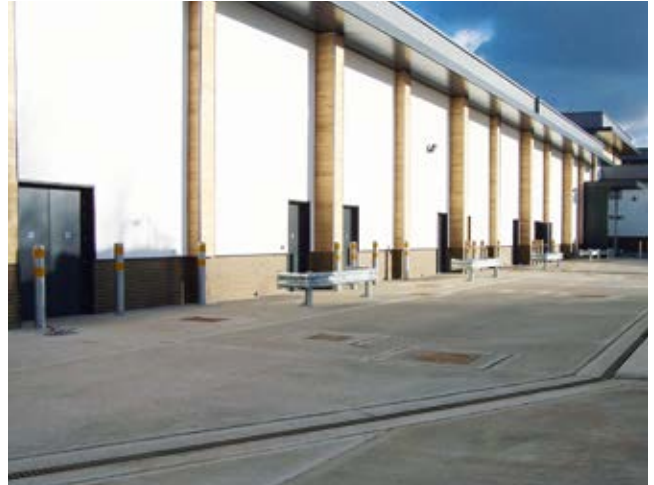
Installation in concrete surface
