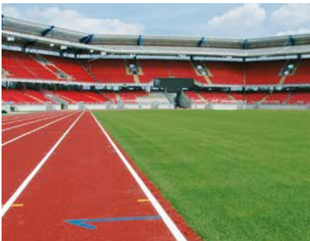
Drainage for running tracks
