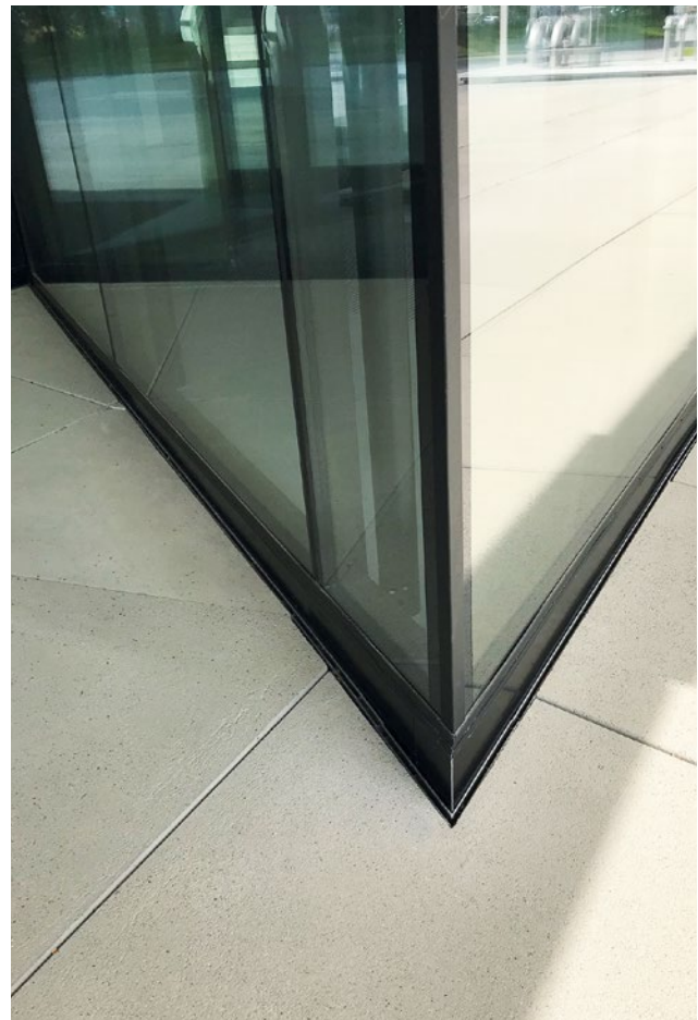
Office building in Müllheim, Germany
