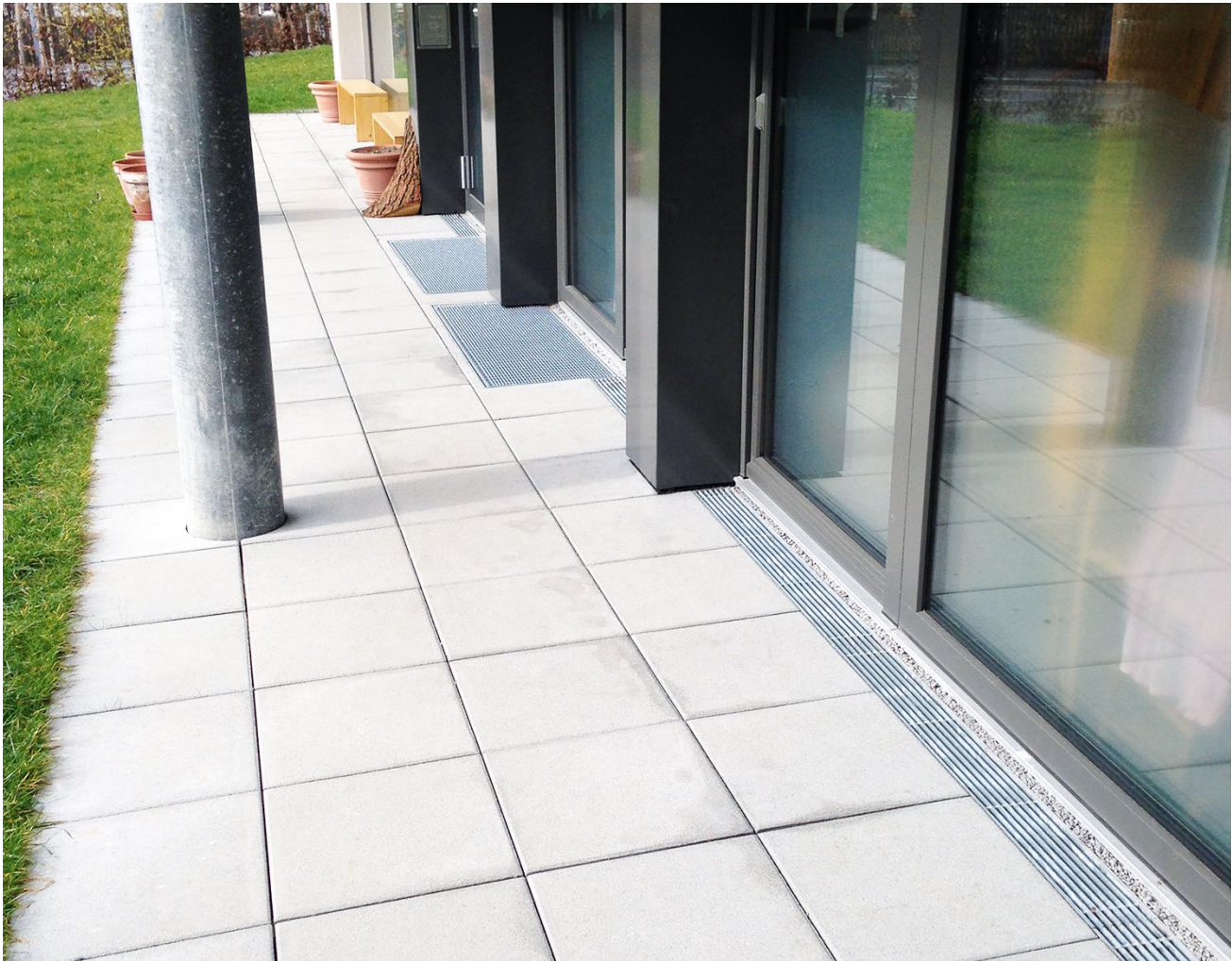
Residence hall Scheuchzerstraße, Zurich, Switzerland
