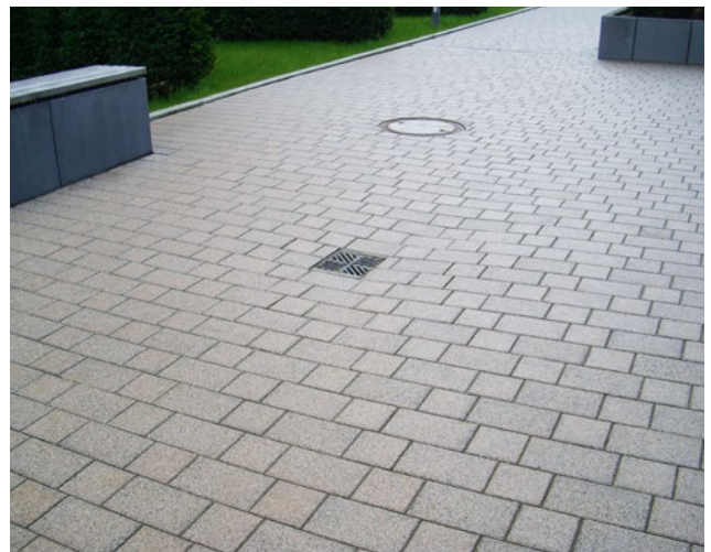
University building in Saarbrücken, Germany
