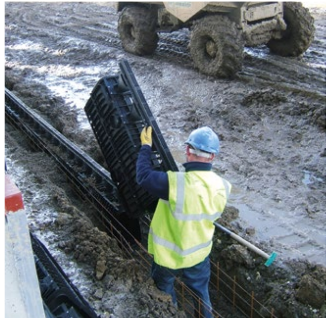
Lightweight elements, installed by one single worker.
