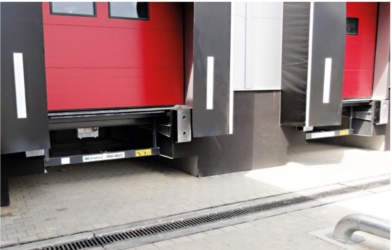
Logistics centre Rossmann, Poland
